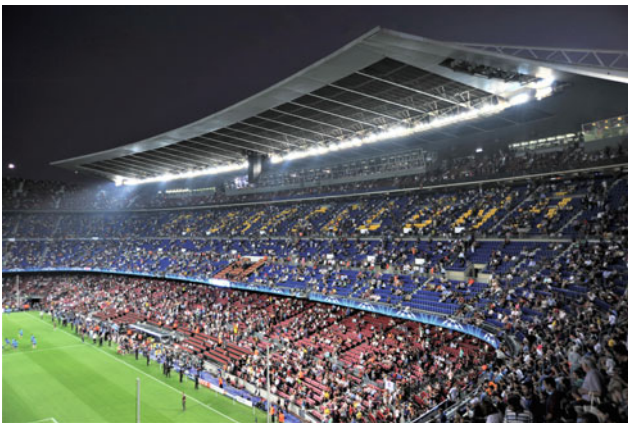
Fig. 78.3 Football pitch lighting. (Image courtesy of Albert Prat)
