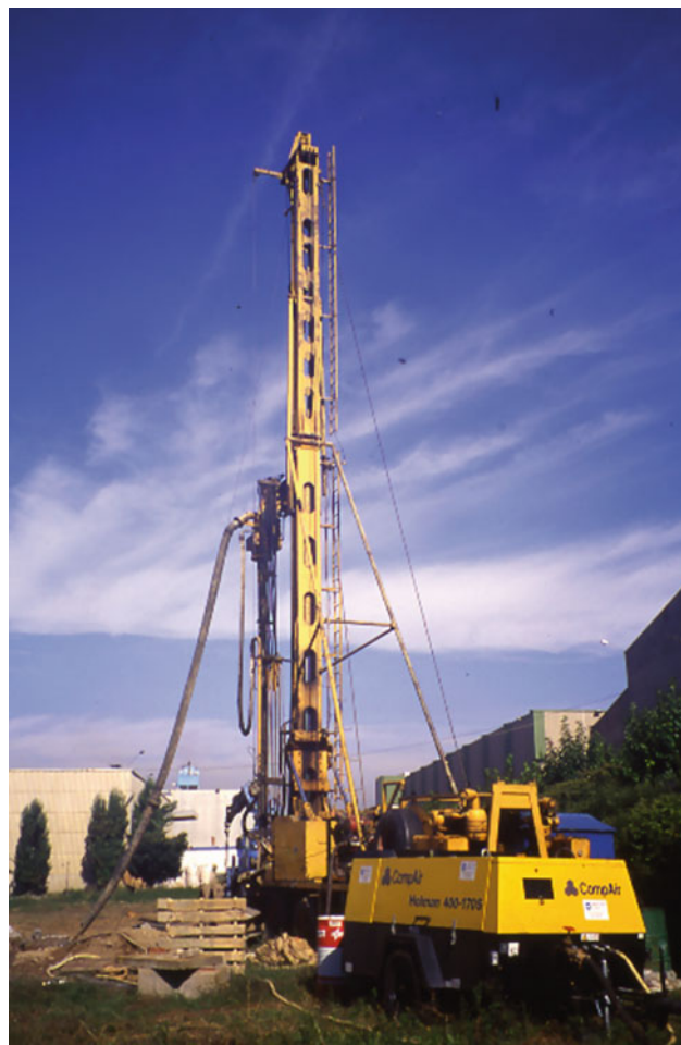
Fig. 5.4 Drilling a water well. (Image courtesy of Raul Osorio)
