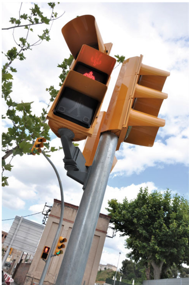
Fig. 63.3 Galvanized steel post for traffic lights. (Photo Joaquim Sanz. MGVM)
