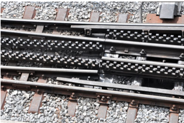
Fig. 32.3 Manganese steel railway tracks (Photo Joaquim Sanz. MGVM)
