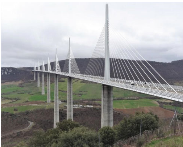
Fig. 36.3 Millau viaduct. (France) (Image courtesy of Xavier Lluís Tartera)
