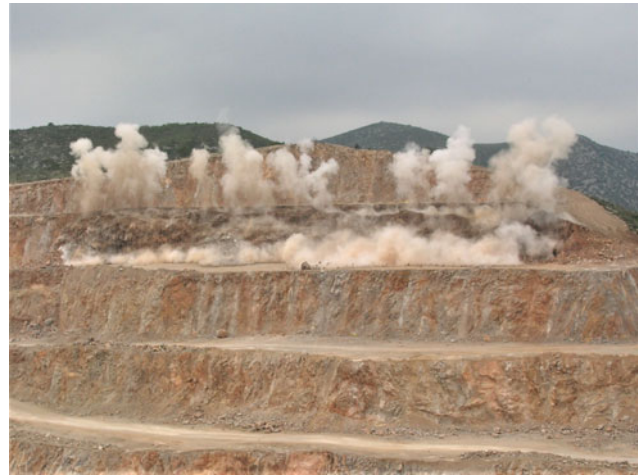
Fig. 81.3 Blasting in a limestone quarry. (Image courtesy of PROMSA)
