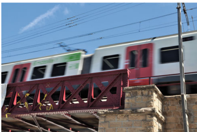
Fig. 28.4 Iron railway bridge (Photo Joaquim Sanz. MGVM)
