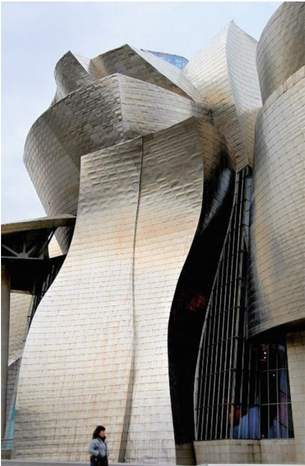
Fig. 59.4 Cladding on the Guggenheim Museum in Bilbao, Spain. (Image courtesy of Joan Clases)
