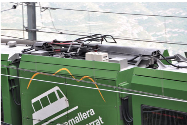
Fig. 49.3 Rack railway catenary. (Photo Joaquim Sanz. MGVM)
