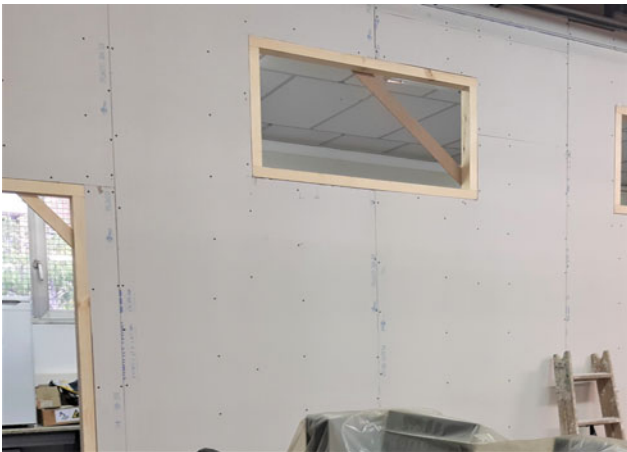
Fig. 89.3 Plasterboard partition. (Image courtesy of Manel Romera)
