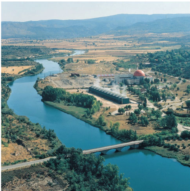
Fig. 61.3 Nuclear power station. (Image courtesy of Javier Castelo)
