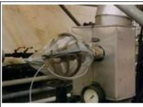
Figure 3.38: Bagging of a leaking valve
