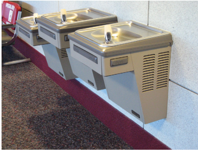
Fig. 8.1.8 These drinking fountains have heat pumps built into them to cool the water. Heat removed from the water, along with heat produced by the heat-pumping process itself, is released into the room air through the louvers visible on the sides of the drinking fountains.
