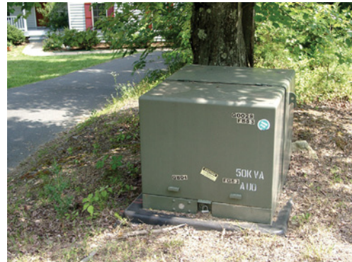
Fig. 11.2.14 This transformer transfers power from a medium-voltage underground circuit to a low-voltage underground circuit used by nearby homes. It handles 50 kV·A or 50,000 W of power.
