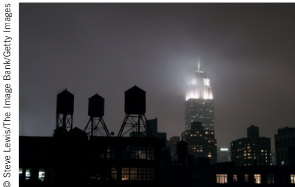
Fig. 5.2.8 Many buildings in New York City have water towers on their roofs. These towers maintain water pressure in the plumbing and help in firefighting.
