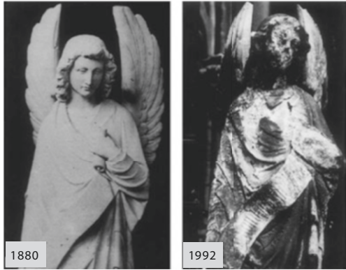
■ Fig. 13.3 Influence of the weathering process on the angel statue at the Peters Portal of Cologne Cathedral. (From Warscheid & Braams, 2000). Cologne, Cathedral, west building, south portal, angel figure, state 1880 © Hohe Domkirche Köln, Dombauhütte. Cologne, Cathedral, west building, south portal, detail view: angel figure, state 1992 © Hohe Domkirche Köln, Dombauhütte
