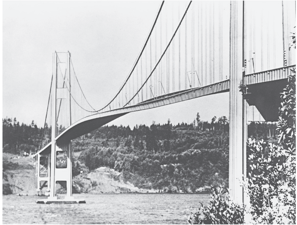
Figure 1.3 The Tacoma Narrows Bridge twisting in the wind. (AP Images)
