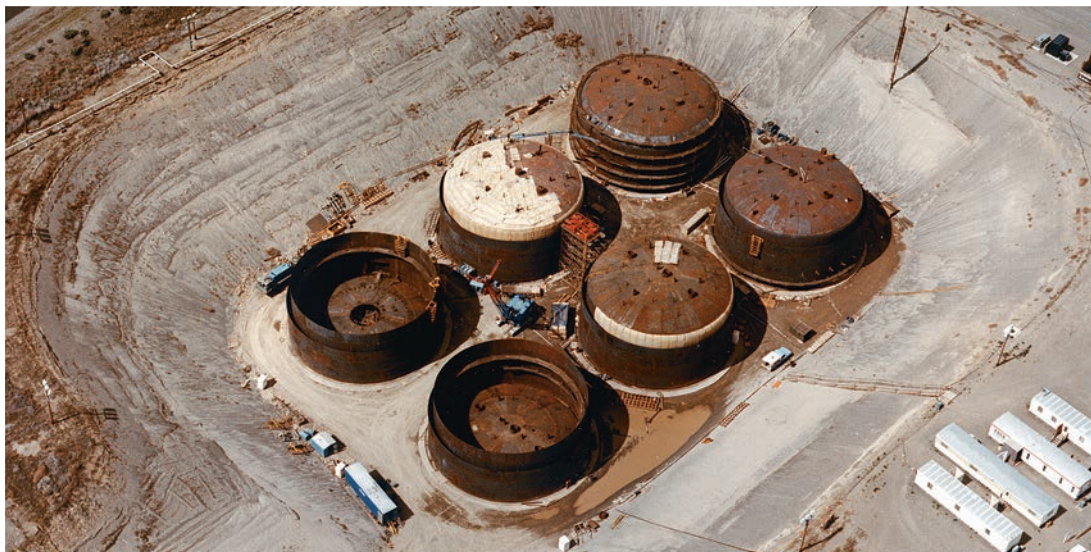
◀ Storage tanks at Hanford, Washington, contain 2.1 \times 10^8 L of high-level nuclear waste. Each tank pictured here holds 4 \times 10^8 L.
