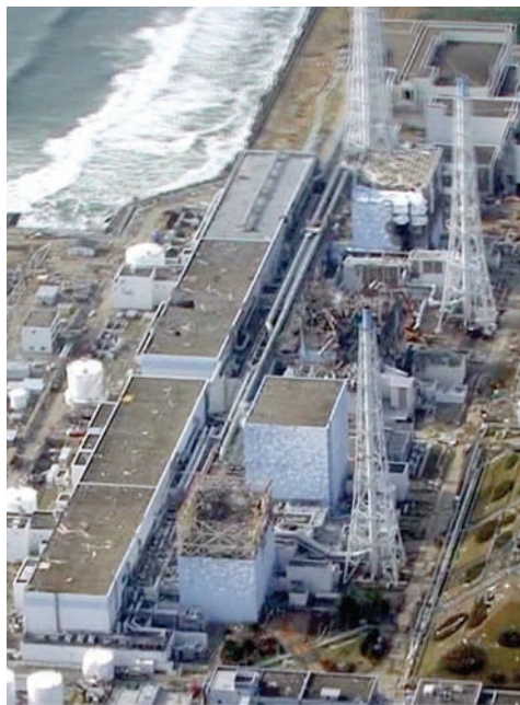
▲ In 2011, the Fukushima Daiichi Nuclear Power Plant in Japan overheated as a result of a 9.0 magnitude earthquake triggered by a tsunami that flooded the coastal plant and caused the cooling system pumps to fail.
