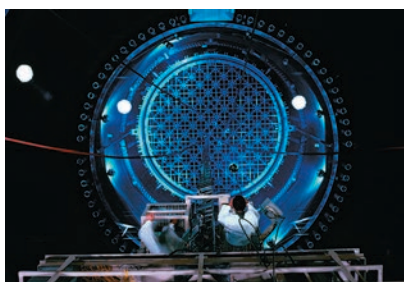
▲ Technicians inspect the core of a nuclear reactor, which houses the fuel rods and control rods.
