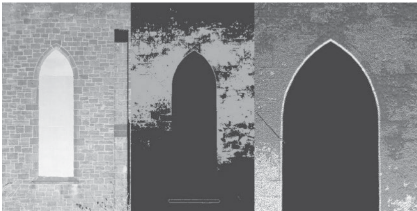
Figure 7.3 Left to right: Point cloud data of wall, section at one specific depth within overall wall surface, “topo” style mapping of entire wall showing various surface levels
