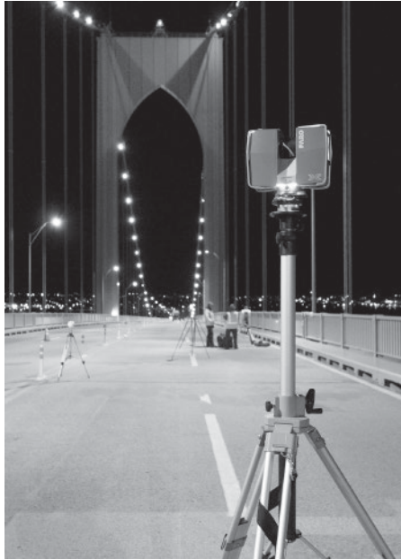
Figure 7.18 Nighttime scanning on bridge using multiple scanners and total station
