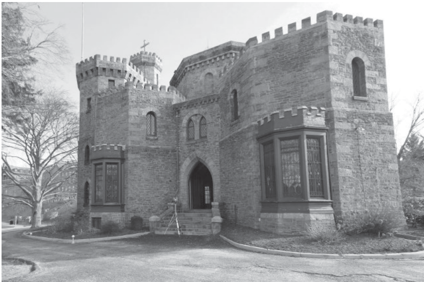
Figure 7.13 LIDAR scanner outside the building; note spherical targets nearby
