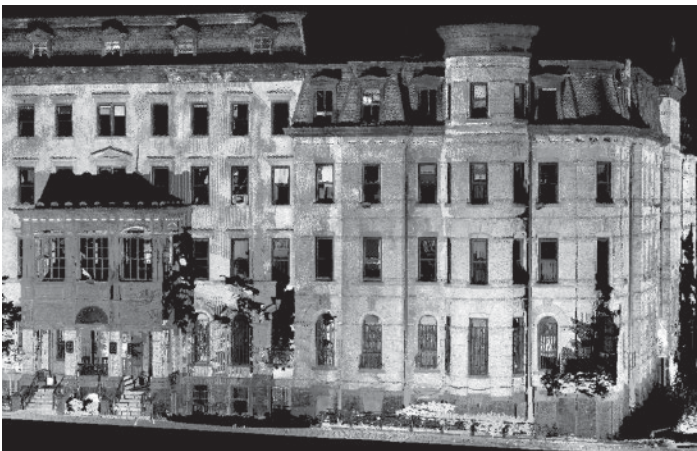
Figure 7.1 Typical view of point cloud data of a building formed by multiple scans at high resolution
