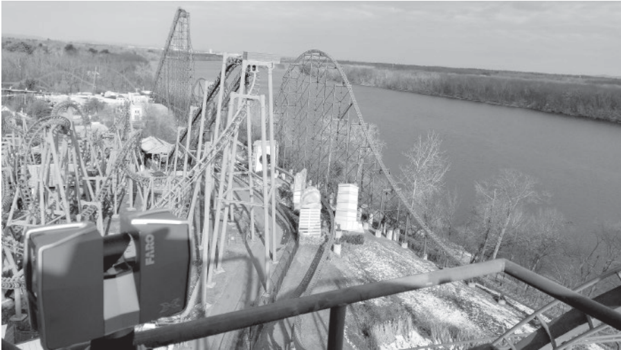
Figure 6.14 Roller coaster being scanned by the FARO lidar scanner
