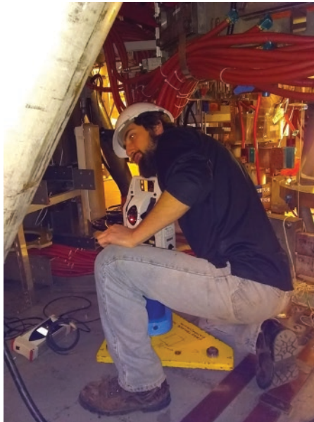
Figure 7.8 Tracker used in close proximity to record surface-mounted CMR data
