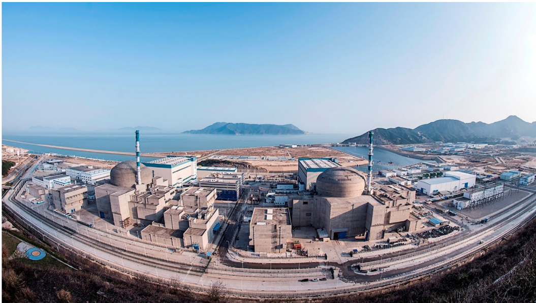
FIG. A1.34 Taishan Nuclear Power Plant, Units 1 & 2, Guangdong, China (year 2020): ( https://www.edfenergy.com/media-centre/news-releases/chinas-second-epr-reactor-taishan-enters-commercial-operation ). Taishan Units 1 and 2 are largest in world nuclear-power reactors. These two reactors based on 1,750-MW el EPR design (net installed capacity is 1,660 MW el , i.e., 90 MW el are used for internal needs (~5% of nominal capacity); NPP gross thermal efficiency – 38% and net – 36%), which were connected to grid in Dec. 2018 and Sept. 2020, respectively. They form part of EUR 8.0 billion (USD 9.7 billion) contract signed by Areva (France) and China General Nuclear Power Group (CGNPG) (China) in Nov. 2007. The EPR design adopted in Taishan was developed by Framatome (France). These EPRs are equipped with Arabelle generators, which are largest single-piece electric generators in world, each weighing 495 tonnes and built by Dongfang Electric. Courtesy and copyright of EDF Energy. Based on: https://www.world-nuclear-news.org/Articles/Chinese-EPR-experiences-performance-issue and https://fr.xco.wiki/wiki/Taishan_Nuclear_Power_Plant
