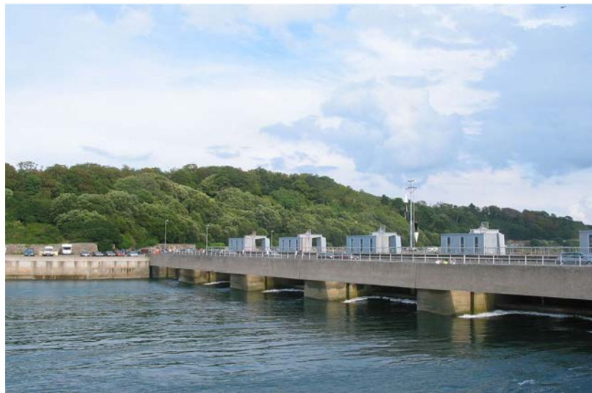
Figure 1.1.44a. Photo of 240\text{-MW}_{\text{el}} Rance tidal power plant ( 10\text{MW}_{\text{el}} \times 24 units)—one of the largest in the world (France). The plant supplies on average 96\text{MW} with a capacity factor of 40\% , providing an annual output of \sim 600\text{GWh} . The barrage is 750\text{-m} long. The plant portion of the dam is 332.5\text{-m} long. The tidal basin measures 22.5\text{km}^2 . Photo taken from Wikimedia Commons, author/username Dani 7C3
