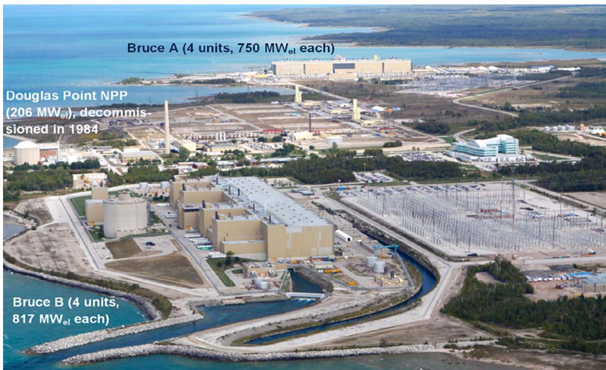
Figure 1.1.15. Aerial view of the largest operating NPP in the world—6384-MW el Bruce NPP. (The Douglas Point NPP was Canada’s first full-scale NPP and the second CANDU reactor. Its success was the major milestone for Canada to enter into the global nuclear-power scene. Construction began on Feb. 1, 1960 and the decommission date: May 4, 1984.) (For more details on all current nuclear-power reactors and plants (layouts, power cycles, diagrams, etc.)—see Appendix A1.) Courtesy of Bruce NPP: www.brucepower.com
