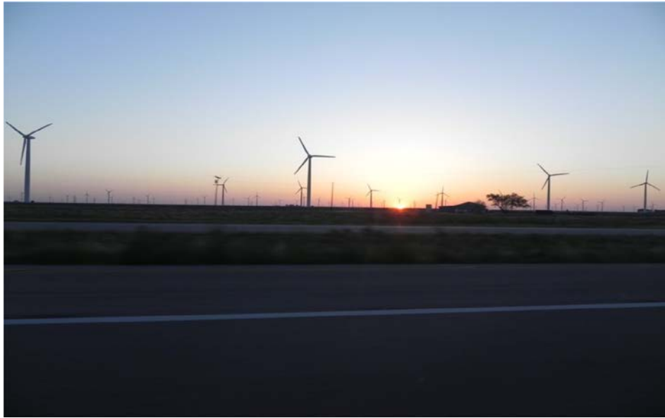
Figure 1.1.23. 781-MW el onshore Roscoe wind-turbine power plant (Texas, USA)—one of the largest in US. Plant equipped with 627 turbines: 406 MHI 1-MW el ; 55 Siemens 2.3-MW el and 166 GE 1.5-MW el . The project cost more than 1 billion dollars, and provides enough power for more than 250,000 average Texan homes and covers a land area of nearly 400 km 2 , which is several times the size of Manhattan, New York, NY, USA. In general, wind power is suitable for harvesting when an average air velocity is at least 6 m/s (21.6 km/h) (It should be noted that the latest and the largest in the world wind turbine by Alstom (6-MW el net wind turbine for the Haliade Offshore Platform has a rotor with the diameter of 150 m and tower 100-m high) can operate within the following range: from 3 m/s (10.8 km/h) and up to 25 m/s (90 km/h) ( http://www.alstom.com/power/renewables/wind/turbines/ )) (see also wind-speed distribution over the US in Figures 1.1.24a and 1.1.24b). Wikimedia Commons, photo by author/username: Fredlyfish4
