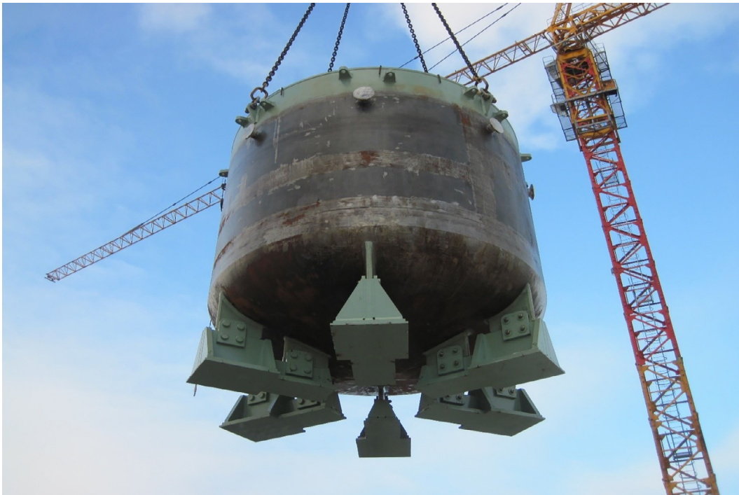
FIG. A1.56 More detailed view of molten-core (corium) catcher for 1100-MW e1 VVER-1200 (Generation-III + ) at Novovoronezh NPP (Generation-III+ reactor's feature): https://www.flickr.com/photos/rosatom/29235111681/in/album-72157672133127091/ . Such catchers can be water cooled or without water cooling. Courtesy of Rosatom
