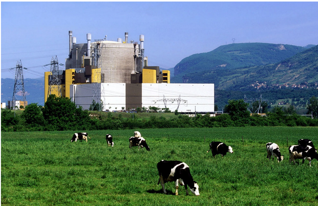
Figure 11.1. View of Superphenix reactor in 1987 ( Guidez and Prele, 2017 )
