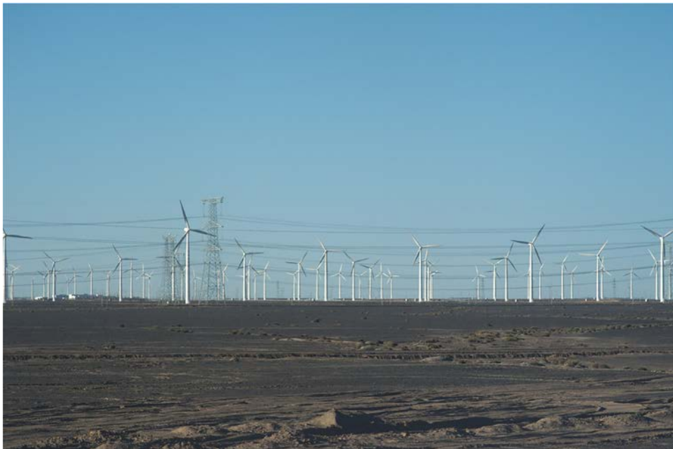
Figure 1.1.21. The world's largest 14,000-MW e1 wind power plant (Gansu, China) ( https://en.wikipedia.org/wiki/Gansu_Wind_Farm ). The total project investment is RMB 120 billion (~$18.6 billion USD). In 2010, the installed wind power capacity in Jiuquan was mainly 200 MW e1 wind farm. The wind farm included 134 wind turbines with a single capacity of 1.5 MW e1 , 11 in each row, 12 rows in total with a row spacing of 900 m at intervals of 300 m. The first 3800-MW e1 phase includes 18 set of 200-MW e1 wind farms and two sets of 100-MW e1 wind farms. The second 8000-MW e1 phase includes 40 sets of 200-MW e1 wind farms. Photo by Popolon: https://commons.wikimedia.org/wiki/File:Guazhou.champs_%C3%A9oliennes.jpg
