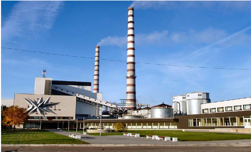
Figure 1.1.12. Photo of the largest in the world 1615-MW e1 Eesti oil-shale-fired power plant (Estonia). The plant equipped with 14 steam generators connected to \sim 230 \text{ MW}_{e1} \times 7 turbines. In 2003, the Unit 8 was reconstructed to use the Circulated Fluidized-Bed Combustion (CFBC) technology, which is more efficient and environmental-friendly (lower SO 2 and CO 2 emissions) compared to the previous technology. Plant has two 251.5-m tall chimneys, which are the tallest chimneys in Estonia. In 2007, the Eesti plant together with the second largest in the world 765-MW e1 Balti oil-shale-fired power plant (so-called, Narva plants) generated about 95% of total power production in Estonia. The oil shale burnt at Narva plants produces about 46% of ash, which is about 4.5 million tons of ash per year. Photo taken from Wikimedia Commons, author A. Simonov. Source: Wikipedia
