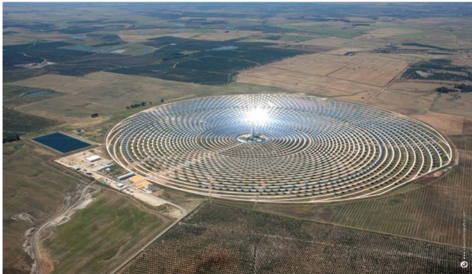
Figure 1.1.28a. Aerial view of the first of such kind Gemasolar—19.9-MW el concentrated solar-power plant with 140-m high tower and molten-salt heat-storage system (Seville, Spain). The plant consists of 2650 heliostats (each 120 m 2 and total reflective area 304,750 m 2 ), covers 1.95 km 2 (195 ha) and produces 110 GWh annually, which equals to 30,000 t/year carbon-dioxide emission savings. This energy is enough to supply 25,000 average Spanish homes, with the storage system allowing the power plant to produce electricity for 15 h without sunlight (at night or on cloudy days). Capacity factor is 63%. Solar-receiver thermal power is 120 MW th , and plant thermal efficiency is about 19%. Molten salt is heated in the solar receiver from 260°C to 565°C by concentrated sun light reflected from all solar-tracking heliostats, and transfers heat in steam generator to water as working fluid in subcritical-pressure Rankine-steam-power cycle. Source: Wikipedia. Courtesy of SENER/TORRESOL ENERGY
