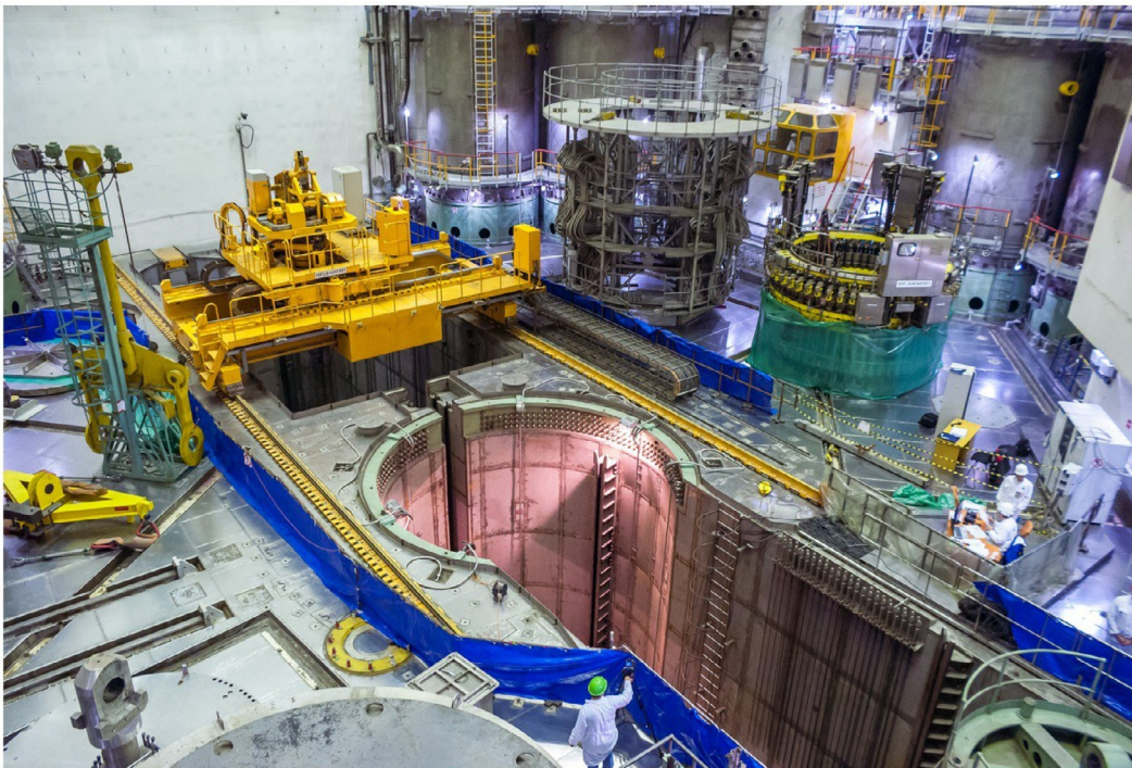
FIG. A1.48 Reactor hall without reactor, 1100-MW el VVER-1200/AES-2006 (Unit 1), Novovoronezh NPP-2. Courtesy of Rosatom: https://www.flickr.com/photos/rosatom/28691689604/in/album-72157672133127091/ ; Photo by R. Pyshkin, 2016
