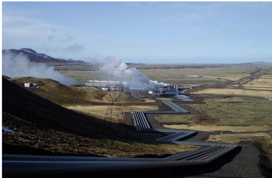
Figure 1.1.38. Aerial view of 303-MW el and 133-MW th Hellisheiði geothermal power plant (45 MW el × 6 units + 33 MW el unit) (Iceland). Photo taken from Wikimedia Commons, original photo from www.thinkgeoenergy.com . Source: Wikipedia
