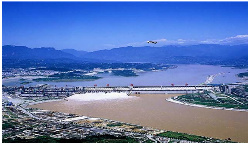
Figure 1.1.16b. Largest in the world by installed capacity (22,500-MW el ) hydroelectric power plant (700 MW el × 30 + 2 × 50 MW el Francis turbines (see Figure 1.1.16c )) (Yangtze River, China). The project costs $32 billion USD (built within 1992–2012) ($ 10 billion USD were used for relocation of people). Height of the gravity dam is 181 m, length—2.335 km, top width—40 m, base width—115 m, flow rate—116,000 m 3 /s, artificial lake capacity—39.3 km 3 , surface area—1045 km 2 , length—600 km, maximum width—1.1 km, normal elevation—175 m, hydraulic head—80.6–113 m. Courtesy of Chinese National Committee on Large Dams. Source: Wikipedia
