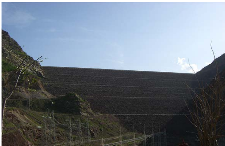
Figure 1.1.17. Photo of the highest in the world 3000-MW el Nurek dam (300 m, Tajikistan). The plant equipped with 335 \text{ MW}_{el} \times 9 = 3015 \text{ MW}_{el} Francis turbines. Photo taken from Wikimedia Commons, author I. Rustamov. Source: Wikipedia
