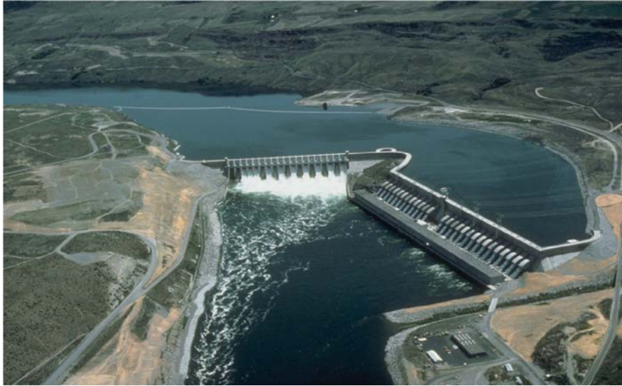
Figure 1.1.19. Aerial view of 2620-MW el run-of-the-river (i.e., an artificial lake upstream the dam is not able to store large amounts of water) Chief Joseph hydroelectric power plant—one of largest in the world (Bridgeport, WA, USA). The plant equipped with 27 Francis turbines \sim 100 MW el each. Height of the gravity dam is 72 m, length—1.817 km, top width—7 m, base width—50 m, flow rate—6030 m 3 /s, artificial lake capacity—0.636 km 3 , surface area—34 km 2 , length—82 km. Photo taken from Wikimedia Commons, original photo by U.S. Army Corps of Engineers. Source: Wikipedia
