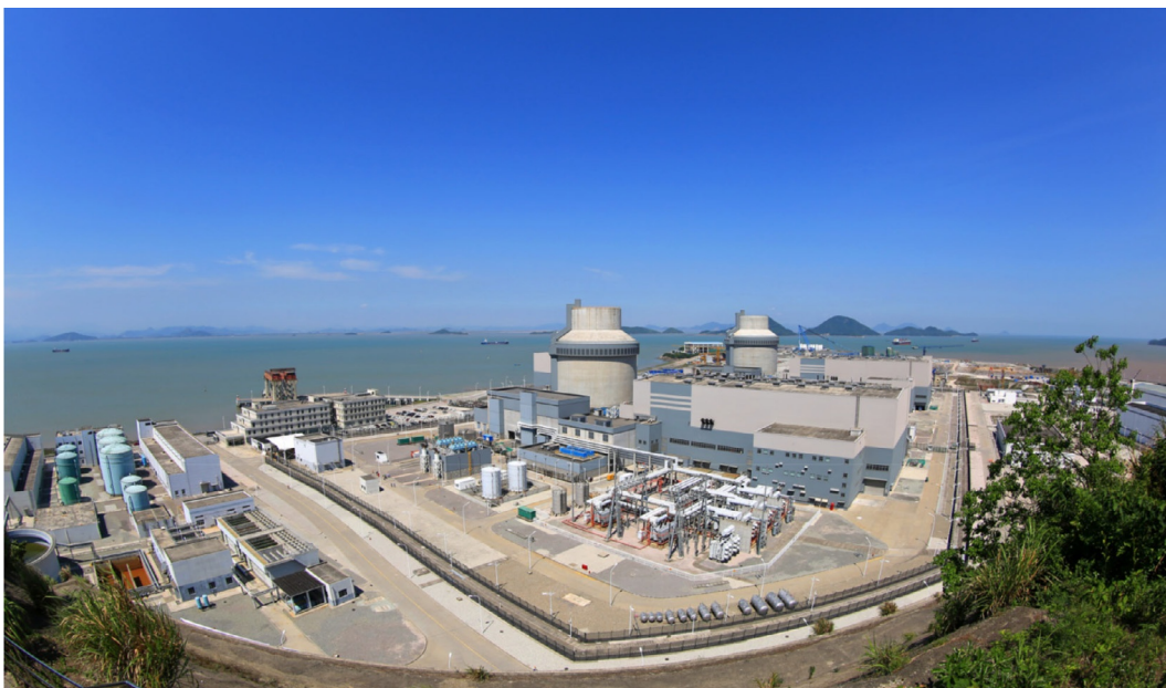
FIG. A1.40 Two 1157-MW e1 AP1000 reactors (Generation-III+) located in two cylindrical-shape containment buildings (commercial operation from 2018) at Sanmen Nuclear Power Plant (Friedman, 2019; ASME J. NERS). Courtesy of Sanmen Nuclear Power Company, Ltd
