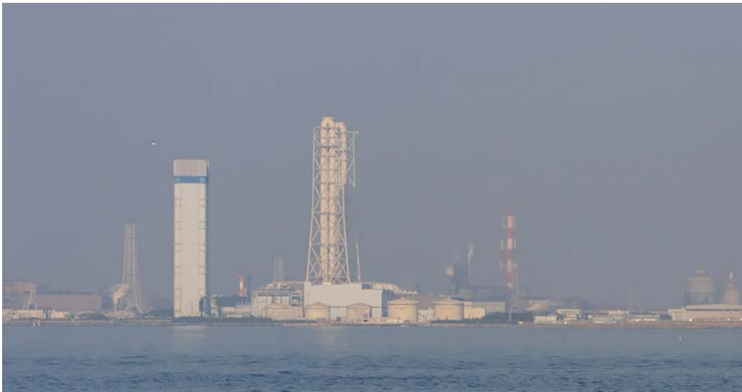
Figure 1.1.11. One of the largest in the world 5040-MW el Futtsu natural-gas-fired combined-cycle power plant (Japan). The plant consists of five generating units: 1520 \text{ MW}_{el} \times 1 + 1000 \text{ MW}_{el} \times 2 + 507 \text{ MW}_{el} \times 2 , and uses Liquefied Natural Gas (LNG). (For more details on combined-cycle gas-fired thermal power plants (layout, power cycle, T - s diagram, etc.)—see Appendix A1.) Photo taken from Wikimedia Commons, author Mr. Hayata. Source: Wikipedia
