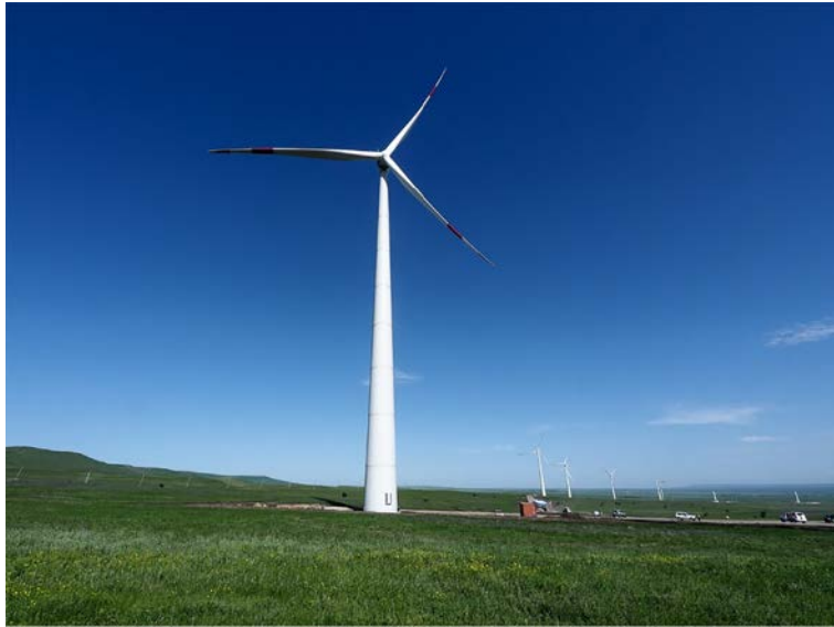
Figure 1.1.22a. Kochubeevskaya Wind Power Plant (Russia). Eighty-four wind turbines by NowaWind (each 2.5\text{MW}_{\text{el}} installed capacity), total 210\text{MW}_{\text{el}} , area 2\text{km}^2 , energy density \sim 105\text{W}/\text{m}^2 ( 105\text{MW}_{\text{el}}/\text{km}^2 ), wind turbine height 150m with rotor, turbine blade 50m and mass 8.6t, tower mass 200t, generator mass 52t, and total mass 320t ( http://novawind.ru/production/our-projects/kochubeyevskaya-wind-farm/ ). Courtesy of Rosatom: https://www.flickr.com/photos/rosatom/50173012221/in/album-72157713699988403/
