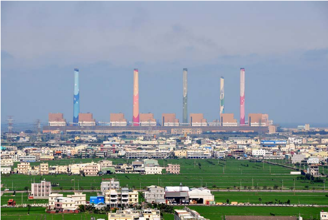
Figure 1.1.9. Aerial view of 5550-MW el Taichung coal-fired power plant (Taiwan)—one of the largest in the world. The plant equipped with 550 MW el × 10 coal-fired steam-generators-turbines + 70 MW el × 4 gas-fired steam generators-turbines and is one of the world’s largest emitters of carbon dioxide with over 40 million tons per year. (For more details on supercritical-pressure coal-fired thermal power plants (layout, power cycle, diagram, etc.)—see Appendix A1.) Photo taken from: https://zh.wikipedia.org/wiki/File:Taichung_Fire_Power_Plant.jpg , author/username Altus. Source: Wikipedia
