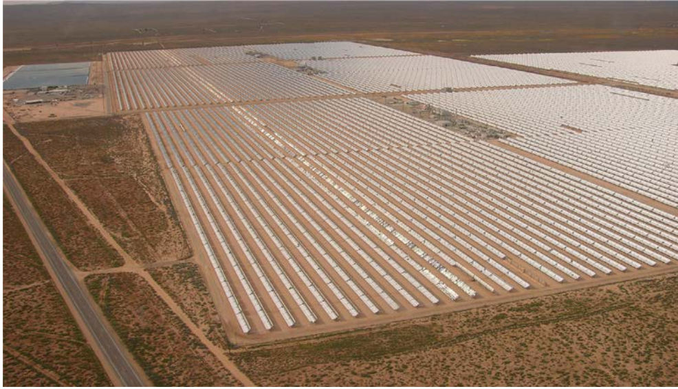
Figure 1.1.29. Aerial view showing portions of Solar Energy Generating Systems (SEGS), California, USA. SEGS is the largest solar-energy power plant in the world consisting of nine concentrated-solar-thermal plants with 354 \text{ MW}_{\text{el}} installed capacity. (See annual average direct normal solar-resource-data distribution over the US in Figure 1.1.27b.) The average gross solar output of SEGS is about 75 \text{ MW}_{\text{el}} (capacity factor is \sim 21\% ), and at night, turbines can be powered by combustion of natural gas. NextEra claims that the SEGS power 232,500 homes and decrease pollution by 3800 t/year (if the electricity had been provided by combustion of oil). The SEGS have 936,384 mirrors, which cover more than 6.5 \text{ km}^2 . If the parabolic mirrors are lined up, would extend over 370 km. In 2002, one of the 30\text{-MW}_{\text{el}} Kramer Junction sites required 90 million dollars to construct, and its O&M costs are about 3 million dollars per year, which result in an initial generating cost of 4.6 \text{ ¢/kWh} , but, with a considered lifetime of 20 years, the O&M and investments interest and depreciation triples the price, to approximately 14 \text{ ¢/kWh} . Wikimedia Commons: Photo by A. Radecki. Source: Wikipedia.
