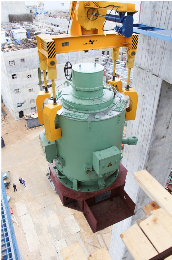
FIG. A1.58 Installation of electrical motor for main circulation pump for 1100-MW el VVER-1200 (Generation-III+), Unit 1, Leningrad NPP (2 units in operation), year 2016: https://www.flickr.com/photos/rosatom/37596923564/in/album-72157668094181020/ . Courtesy of Rosatom
