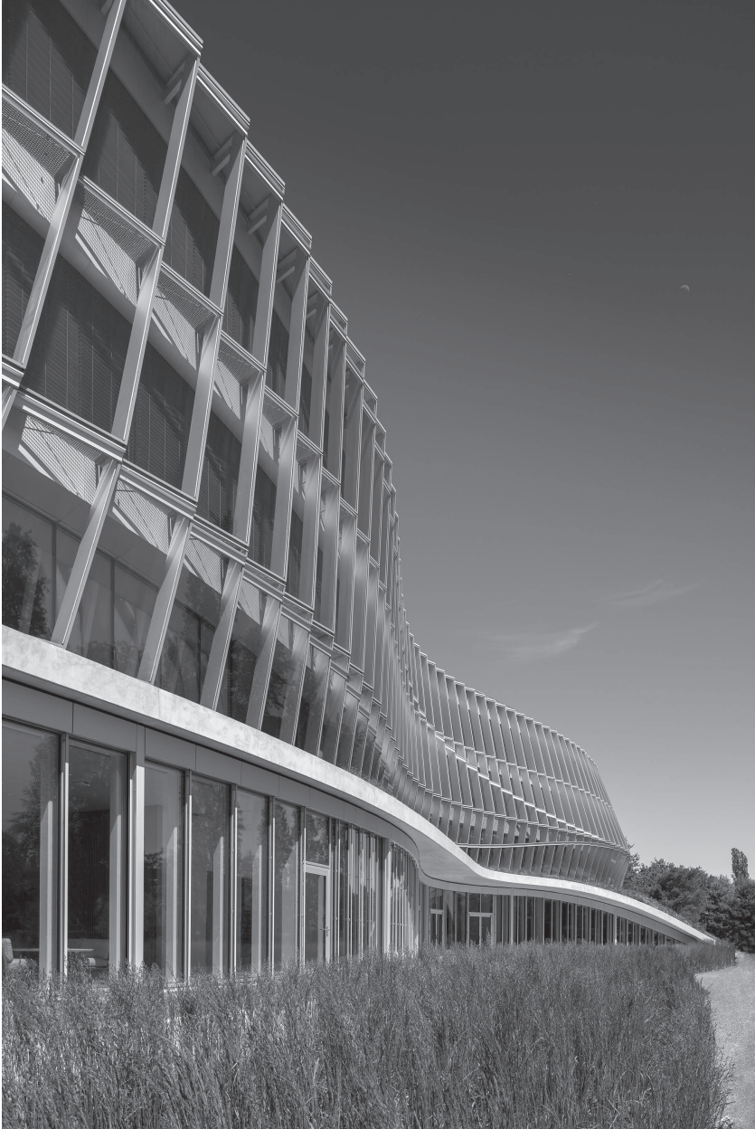
FIGURE 4.6 Photo, International Olympic Committee (IOC) Headquarters, Switzerland, 3XN, 2019
