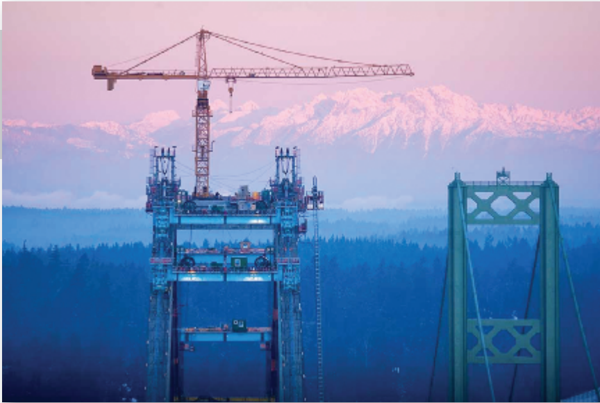
Courtesy of Bechtel Corporation
