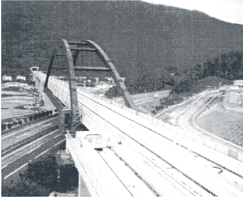
Figure 6.12 Yamanashi Maglev Test Line: Ogatayama Bridge over the Chuo Expressway. Courtesy of Central Japan Railway Company and Railway Technical Research Institute , Tokyo, Japan.
