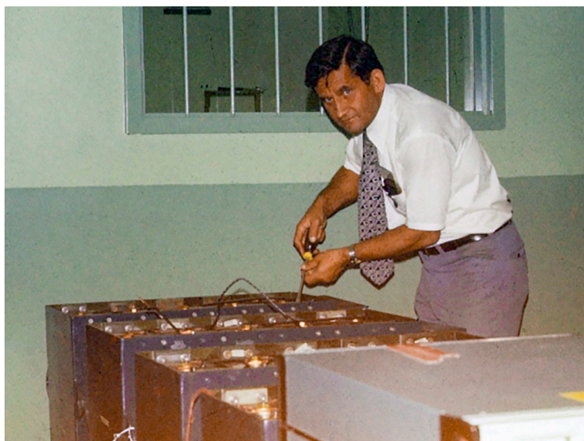
Nikola Marincic of Battery Engineering Inc. built the first preproduction rechargeable lithium cells at a converted truck garage in Boston, Massachusetts. (PHOTO COURTESY OF LIDIJA ORTLOFF.)
