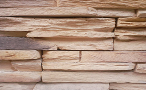
Figure 5.17 An example of a complex wall surface
