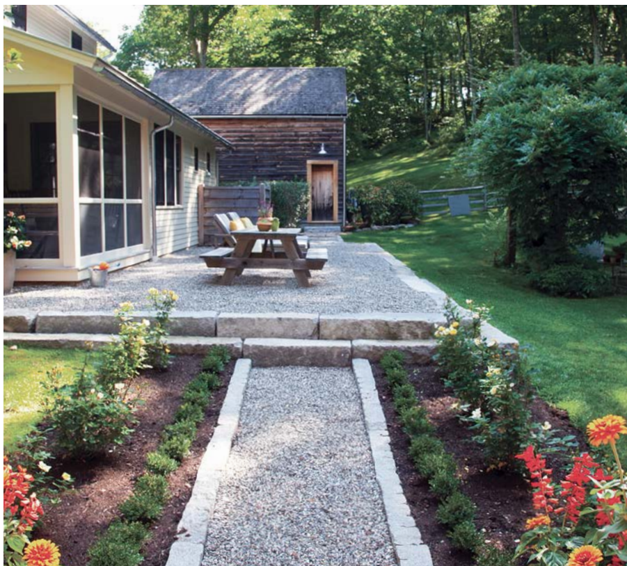
above • Granite cobbles hold in pebbles both along a path and around a terrace, on which a simple picnic table rests for outdoor dining.
