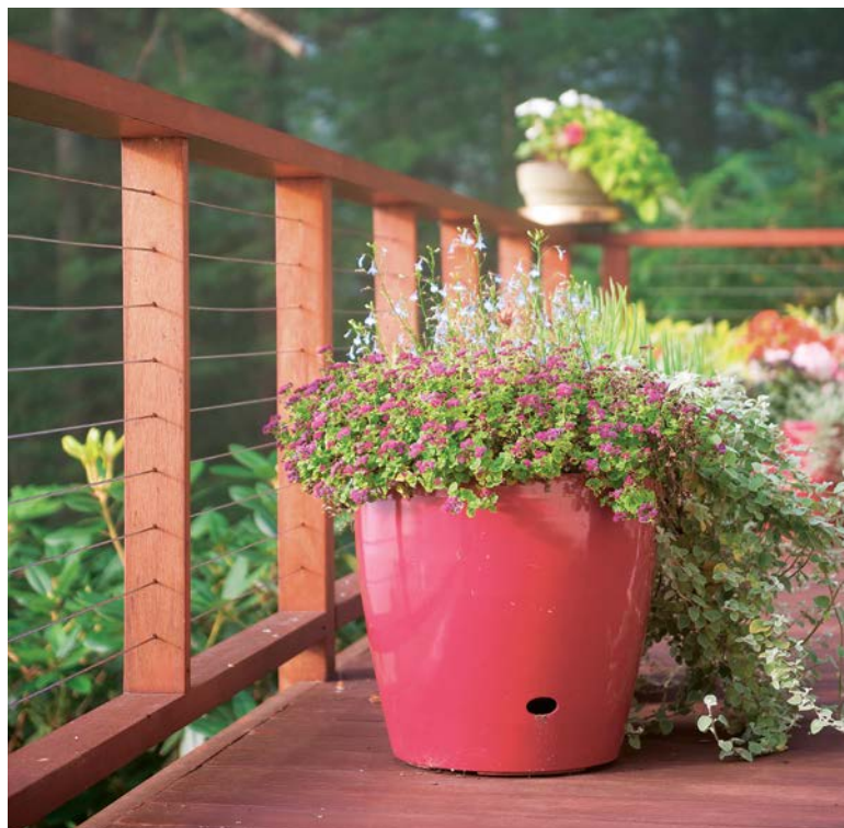
above • A mahogany framework supports stainless-steel cables that meet the building code while allowing a view of the landscape beyond. A lightweight resin pot cast with a watering hole allows for watering with a hose without disturbing the blossoms.
