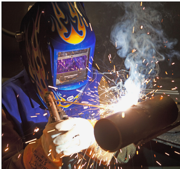
FIGURE 14-1: Steel pipe being stick welded.
