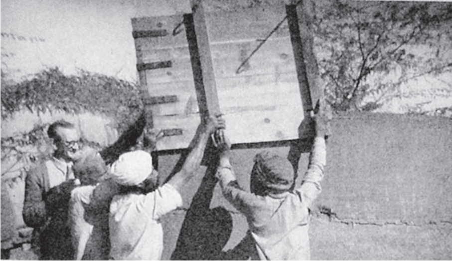
FIGURE 2.20. George Middleton helping construction workers remove the mold he designed for rammed earth wall construction. Source: "Decent Housing at Low Cost: New Delhi's International Exhibition," United Nations Bulletin 16, no. 5 (1954): 187.
