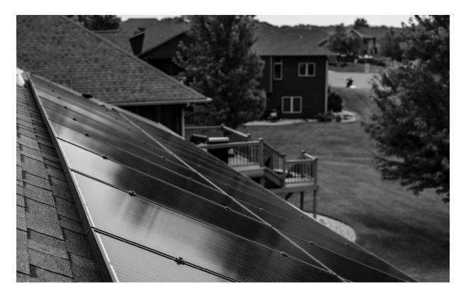
Grid-tied systems are connected to the public electricity grid and do not require a battery for storage. When your gridtied solar system produces more electricity than you can use, the excess is sent back into the power grid. Depending on the net metering policies in your area, you may get credit for this excess electricity.
