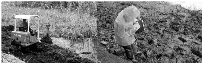
Figure 2: Canal being dredged to create a 3.5 m raised platform within the canal, with double rows of planted trees.
