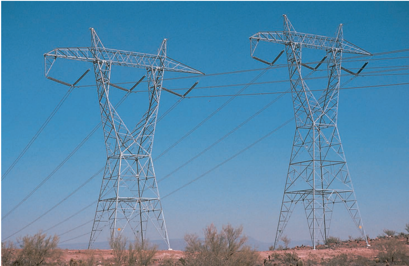
FIGURE 6.13 What is the nature of the electric current carried by these conducting lines? It is an electric field that moves at nearly the speed of light. The field causes a net motion of electrons that constitutes a flow of charge, a current. Source: © Arizona Public Service Company.
