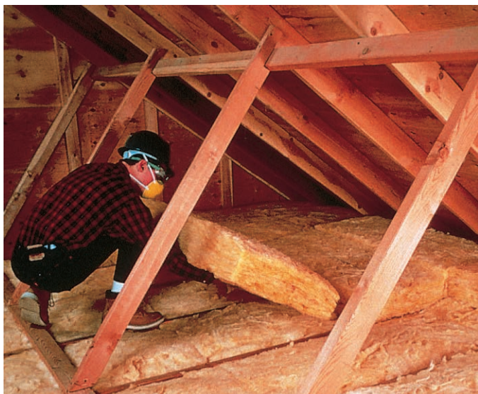
FIGURE 4.14 Fiberglass insulation is rated in terms of the R-value, a ratio of the conductivity of the material to its thickness.
