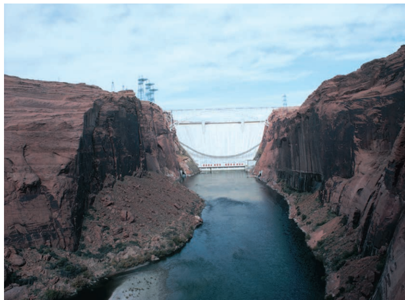
FIGURE 3.1 This is Glen Canyon Dam on the Colorado River between Utah and Arizona. The 216 m (about 710 ft) wall of concrete holds Lake Powell, which is 170 m (about 560 ft) deep at the dam when full. Water falls through 5 m (about 15 ft) diameter penstocks to generators at the bottom of the dam. Source: © Bill W. Tillery.
