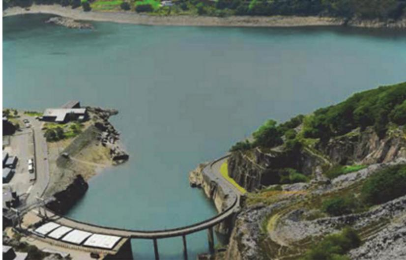
**Figure 3.1C:** Dinorwig pumped hydro asset is the fastest power generation unit in Wales, UK, with the ability to deliver 1.7GW in 16 seconds.
