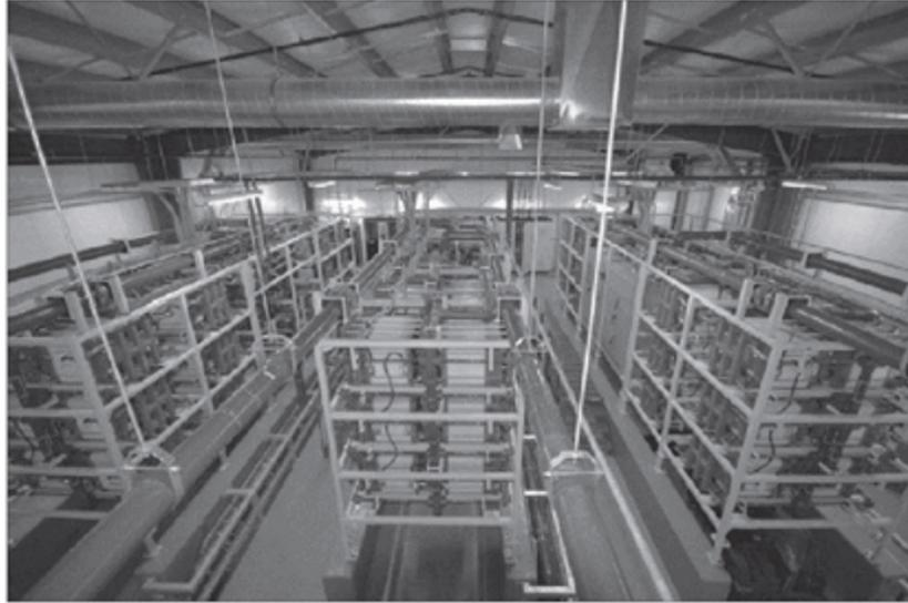
**Figure 4.16b:** Prudent Energy installed 600kW/3,600-kWh VRB-energy storage system at Gills Onions, Oxnard, CA.
