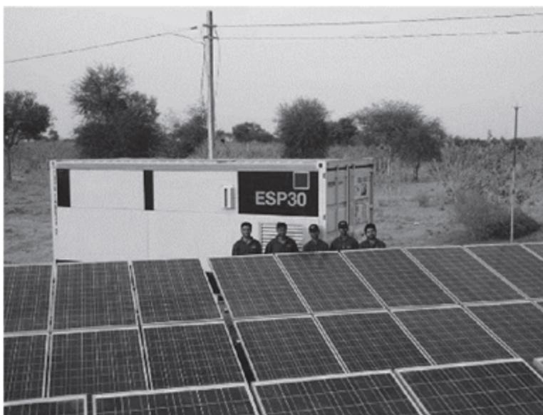
**Figure 4.18b:** Solar power generation plant combined with storage facility with RFBs. Credit: [238].
