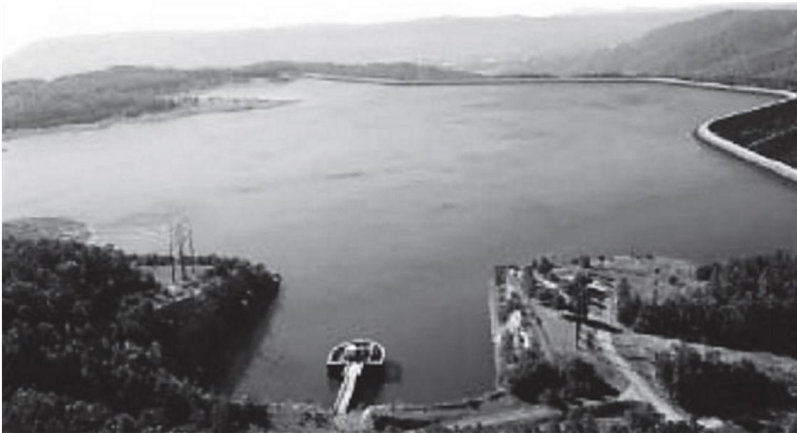
**Figure 3.1B:** Man-made Upper Reservoir of Tennessee Valley Authority's Raccoon Mountain PH Plant: the facility can generate 1620 MW for up to 22 hours [7].
