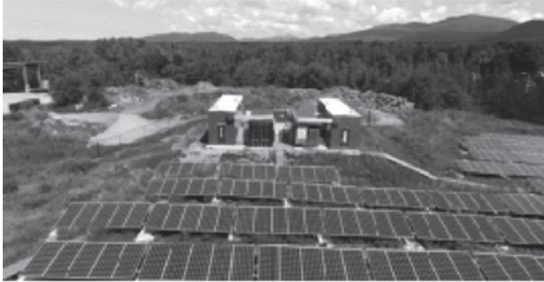
**Figure 4.3:** Stafford Hill Solar Farm (2.3 MW) and battery system (4 MW/ 3.4 MWh) in Rutland, VT; Photo: Green Mountain Power (Source: [32]).
