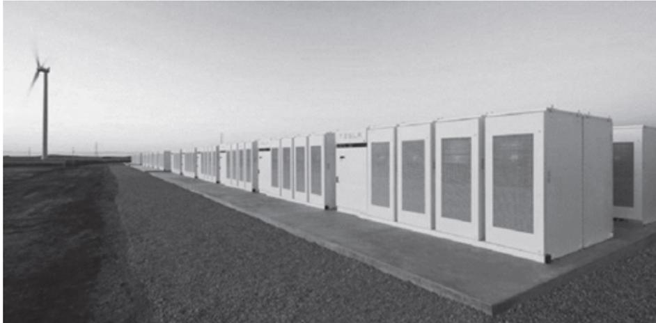
The Hornsdale Power Reserve, a 100 MW battery storage facility in South Australia. Credit: Tesla
