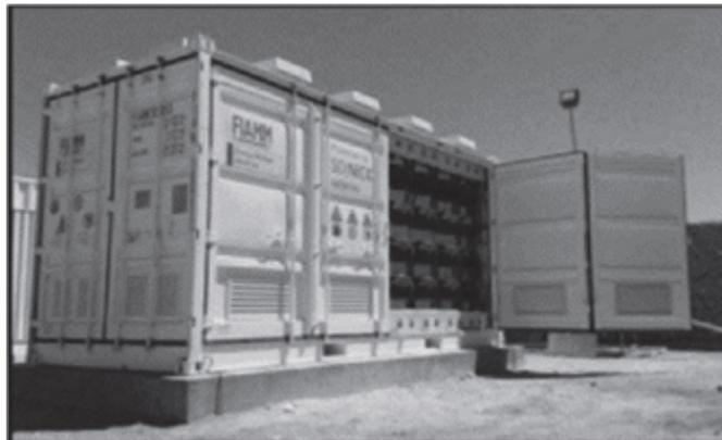
**Figure 4.12c:** An FZSoNick Na-NiCl<sub>2</sub> battery system supporting the integration of renewable remote photovoltaic energy in South America.
