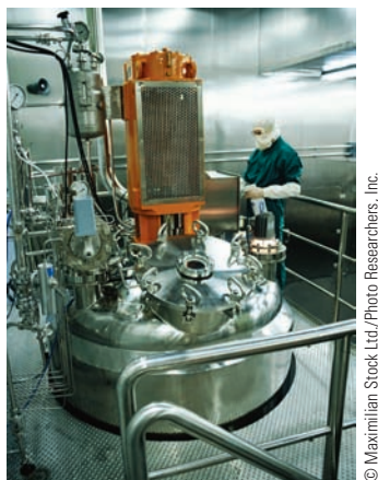
FIGURE 7.38 Fermentation tanks used in modern penicillin production.
