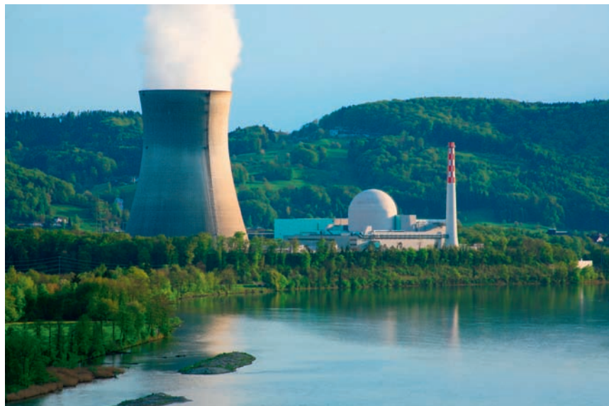
FIGURE 19.9 A nuclear power plant. The large structure on the left is a cooling tower; the containment building is the smaller building on the right with the domed top.
