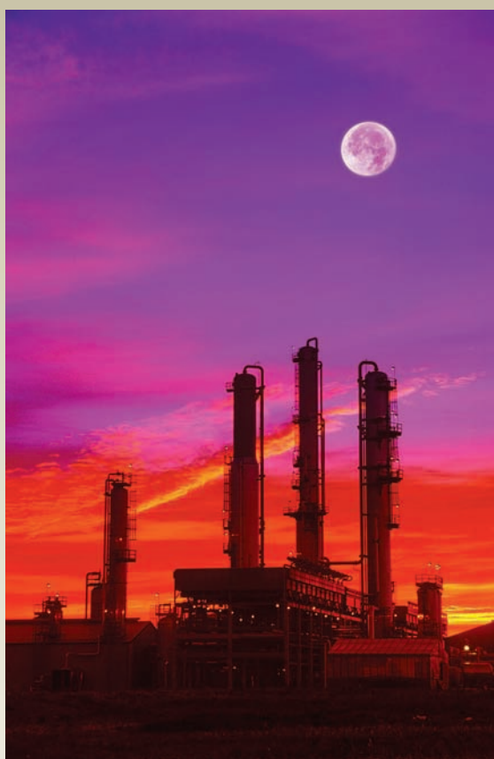
A petroleum refining tower.
