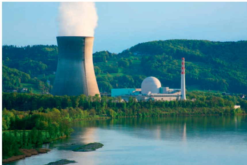
FIGURE 19.9 A nuclear power plant. The large structure on the left is a cooling tower; the containment building is the smaller building on the right with the domed top.
