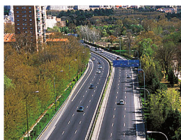
la autopista lah aootopeestah highway/expressway
