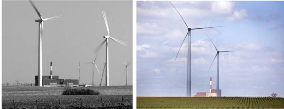
FIGURE 2.10 Symbiotic coupling of nuclear and wind technologies views during winter and summer. The two units 2309 MWe Boiling Water Reactors LaSalle nuclear power plant near Marseilles, Illinois, United States operated by Exelon Nuclear corporation and the Grand Ridge Wind Farm operated by Invenery LLC in the adjacent farmland near Ransom in Illinois, United States. The nuclear reactor and the wind turbines are both manufactured by the General Electric Company [6].
