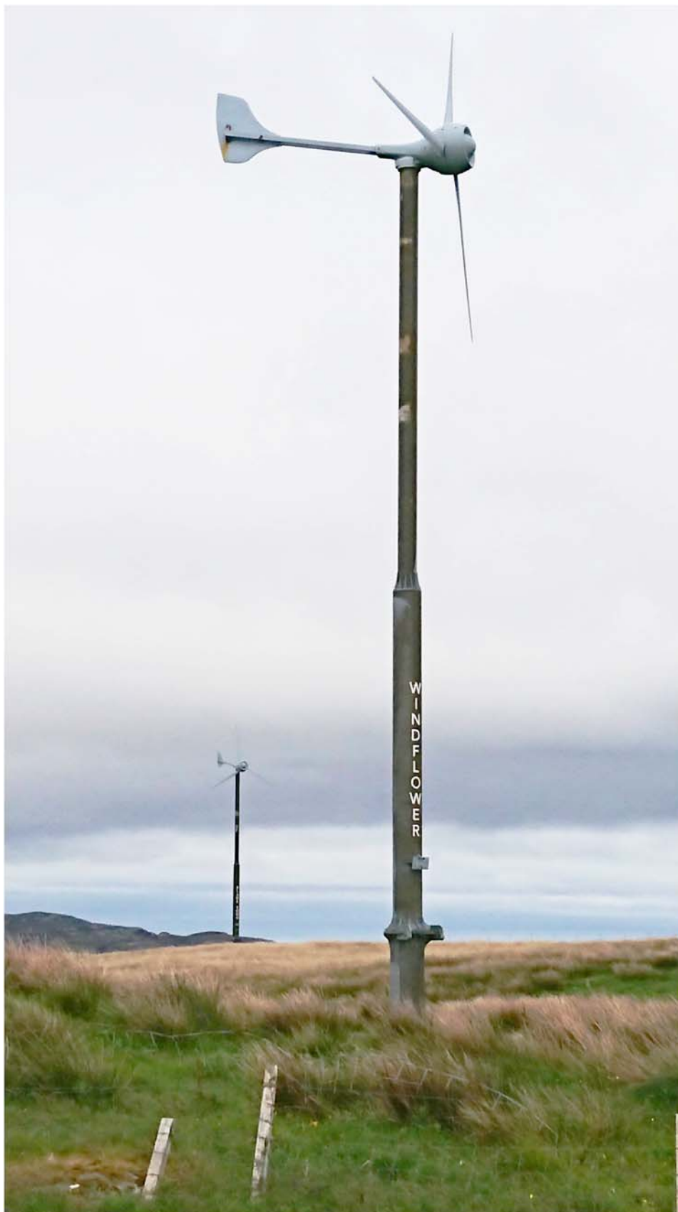
FIGURE 30.17 Wind Flower and Blade Song are two named turbines on North Uist, Scotland. Photo: B Dower. All rights reserved.
