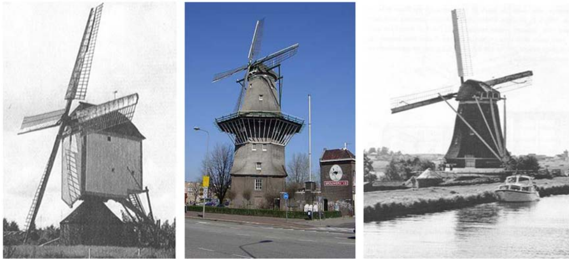
FIGURE 2.7 Evolution of Dutch windmill designs: rotating cage post windmill with rotating lever wheel in the back and pegged wheel acted as a yaw mechanism to rotate the windmill to face the wind ( left ), tower design (Funenkade Olen windmill, Amsterdam, Holland) ( center ), and rotating-roof smock design for pumping drainage water ( right ).
