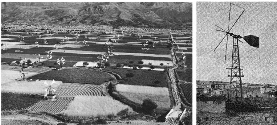
FIGURE 2.5 Sail water-pumping windmills harvesting the wind in large numbers on the island of Crete in the Mediterranean Sea.
