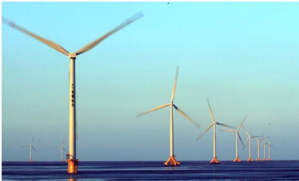
FIGURE 10.16 Different types of support structures for a wind farm in China.
