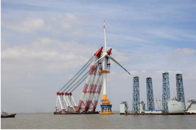
FIGURE 12.8 Installation of the wind turbine in China.
