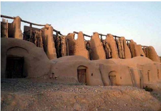
FIGURE 2.3 Remaining vestiges of ancient vertical-axis windmills or “Panemones” at Seistan, near the border between Iran and Afghanistan. The rotors were made from cloth or bundles of reeds and wood.
