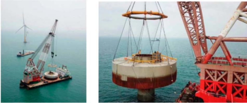
FIGURE 25.4 Concrete caisson or monopile suction caisson.
