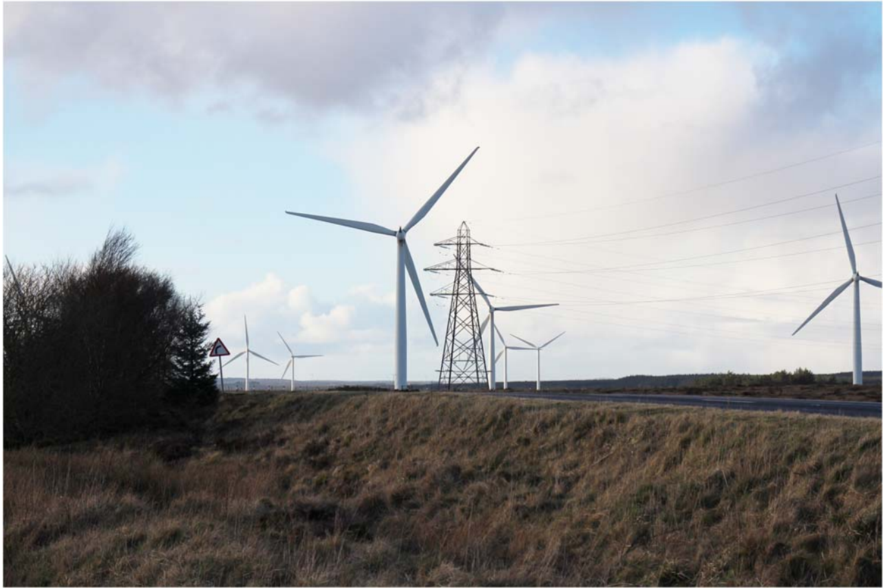
FIGURE 30.11 The height and size of these turbines is difficult to estimate despite the presence of clear scale indicators such as trees and pylons. Photo: B Dower. All rights reserved.
