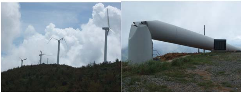
FIGURE 12.11 Damages to blades and tower due to hurricane Saomai.
