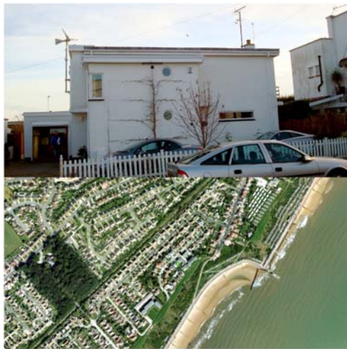
FIGURE 9.20 Windsave WS1000 turbine ( t ) and ultrasonic anemometer (Vaisala WMT50, a ) on house in the coastal town of Felixstowe. Measured wind-speed data, March 2008–February 2009. Average wind-speed is 2.83 m/s. NOABL wind-speed is 5.7 m/s, and for NOABL-MCS (2010), 2.2 m/s.
