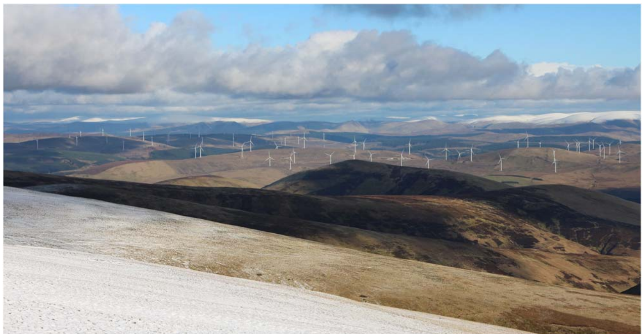
FIGURE 30.22 An informal layout in rolling upland, Clyde Wind Farm, UK. Photo: B Dower. All rights reserved.
