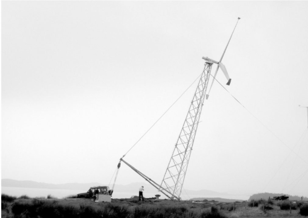
Figure 9.27 Winch erection of a 50 kW wind turbine. Winch loading is highest at the start of the lift when the weight moment is greatest; once near the vertical, the winch load reduces almost to zero: the back stay seen on the right will shortly take up the load. (Photo courtesy Paul Pynn)
