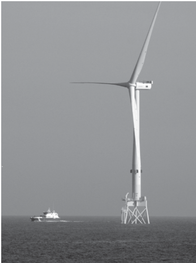
Figure 1.2 Thirty years' growth: (a) the 'Californian wind rush', San Geronio, 1986; (b) Vestas 8 MW wind turbine in the Aberdeen Offshore Array, 2018: this single machine has a greater power output than all the wind turbines in the top picture combined.
