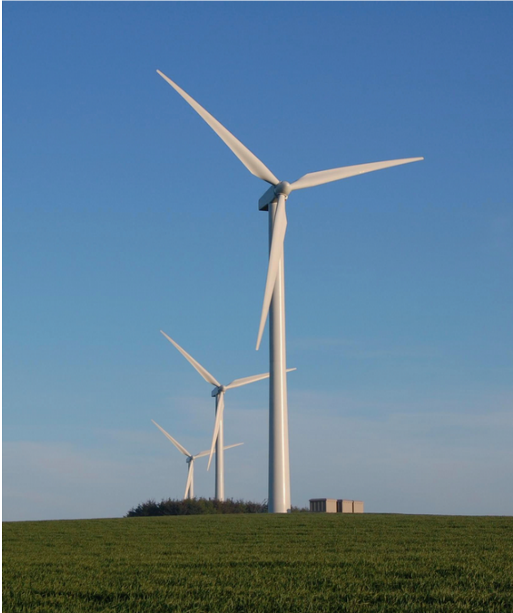
Figure 3.21 All lined up. Measurements from this linear array of Vestas V52s (4.4D spacing) illustrate the properties of rotor wakes. Figure 3.20 shows wake velocity profiles, while Figure 9.6 shows the influence of wind direction on wake power deficits. (Balquhindachy windfarm, Aberdeenshire: photo reproduced with kind permission of Greenspan Energy Ltd)
