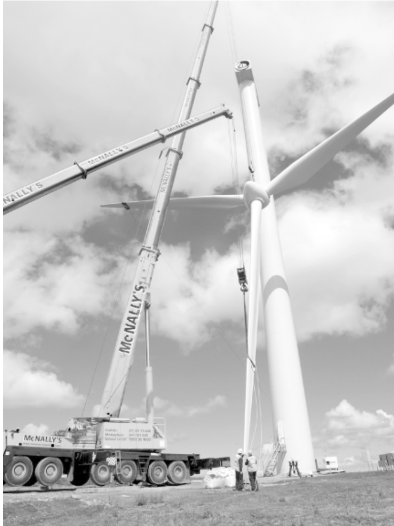
Figure 9.26 Main rotor lift for a Vestas V52. A tailing crane (out of picture) is steadying the rotor. Single-crane rotor lift is also possible using a proprietary turning mechanism under the crane hook.
