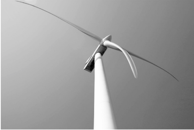
Figure 3.8 Highly loaded rotor. In normal operation, the axial thrust loading is much greater than the tangential and causes the visible downwind bending of the blades. (Courtesy Vestas Wind Systems A/S)
