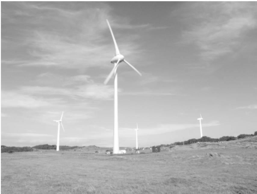
Figure 11.12 The Isle of Gigha Community windfarm today. The original project of three second-hand V27s was commissioned in 2004, with a fourth turbine (Enercon E33 in foreground) added in 2013.
