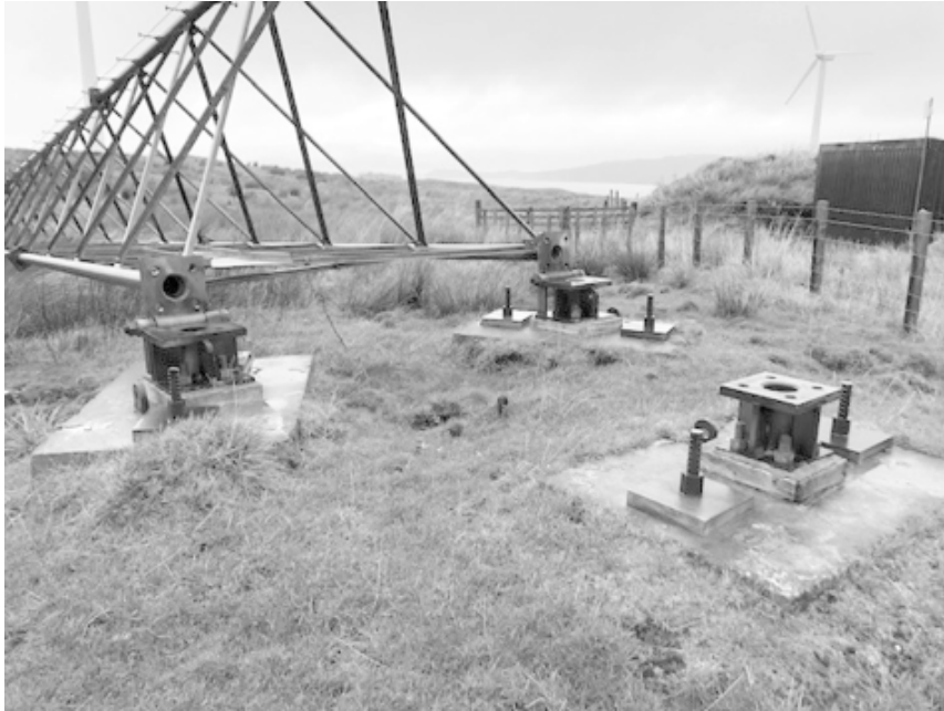
Figure 9.19 Hybrid rock anchor foundations. Each leg of the hinged lattice tower attaches to an individual reinforced concrete plinth, which is pinned to bedrock by two 6 m rock anchors. Demonstration project on the Island of Luing, Scotland. (Photo courtesy Shane Cadzow)
