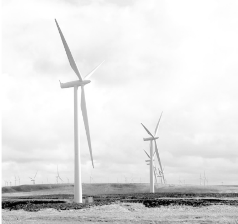
Figure 4.12 Parked rotors. These machines are stopped with their blades fully pitched to 90^\circ in the braking position. (Siemens 2.3 MW turbines at Whitelee windfarm)
