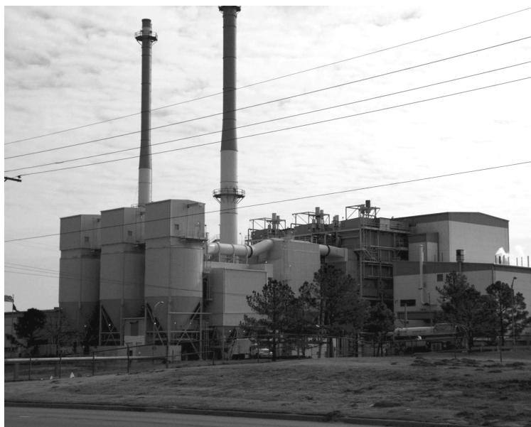
FIGURE 53.18 (a) Schematic and (b) photo of a waste incineration plant. (Source: Baukal, C. E. (ed.) 2003. The Handbook of Industrial Burners , CRC Press, Boca Raton, FL.)
