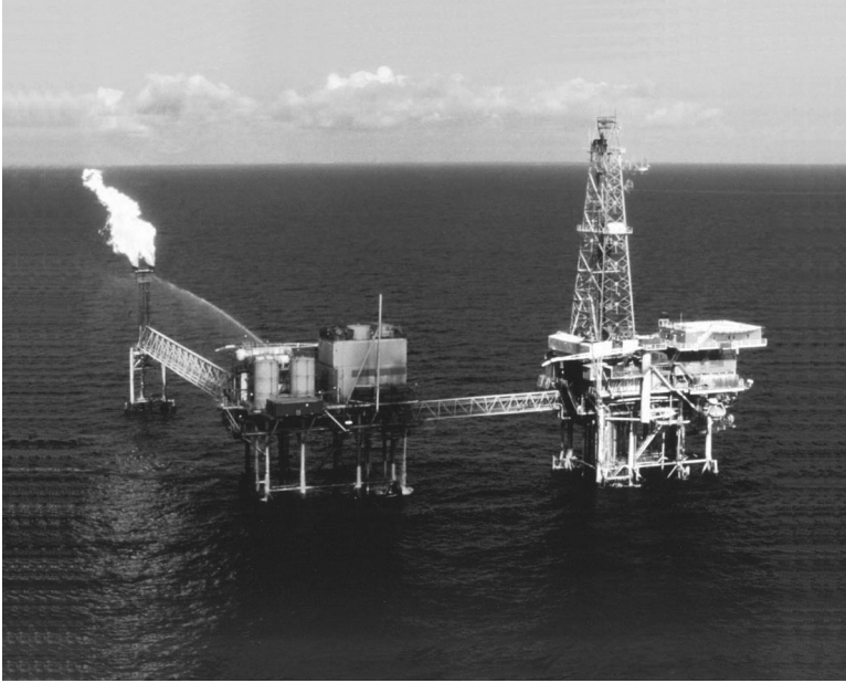
FIGURE 53.7 Flare on an offshore oil platform (courtesy of John Zink Co., Tulsa, OK).
