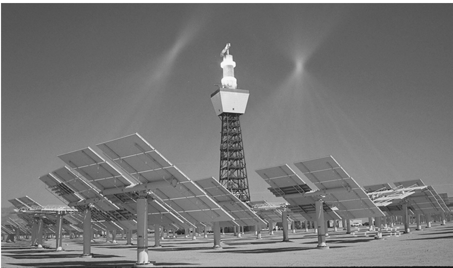
FIGURE 67.2 Warming the receiver at Solar 2 in Dagget, CA. The “wings” one either side of the receiver result from atmospheric scattering of the sunlight reflected from the heliostat field. (Photograph courtesy of Sandia National Laboratories.)
