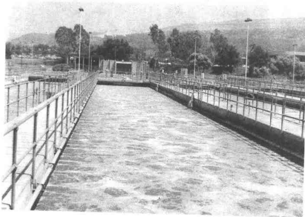
FIGURE 7.16 Plug flow activated sludge process.
