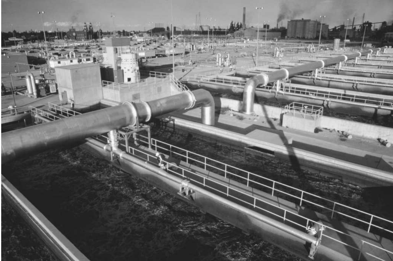
A wastewater treatment plant in Detroit, Michigan.
